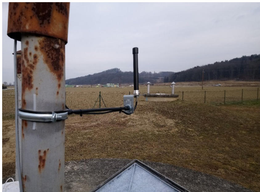
Figure 10 Mounting of the high gain antenna.
